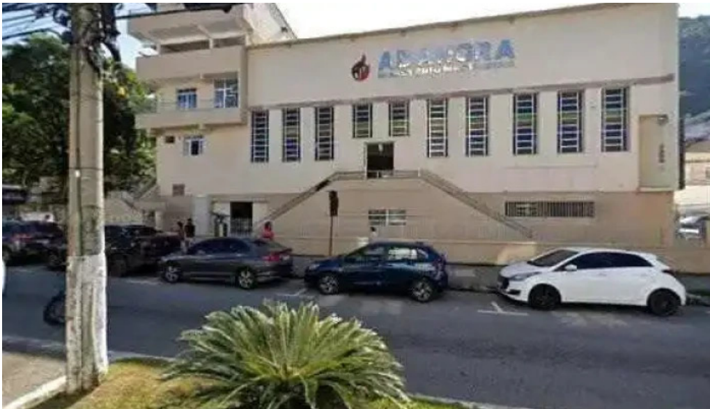
Droga raia street view e 360deg
