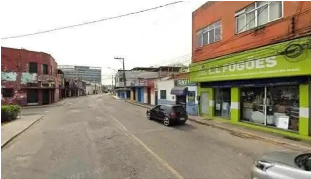
Droga raia street view e 360deg
